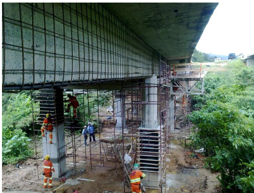
Figure 2. Reinforcement of beam joists under construction on BR-116 / SP.
