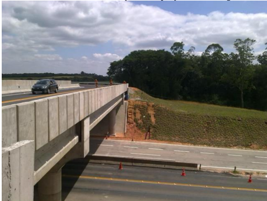
Figure 1. Viaduct built on the SP300 Road.
